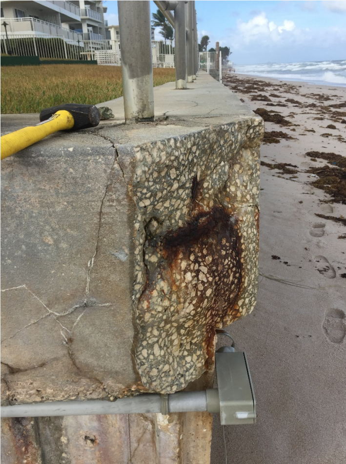
South Florida Seawall
