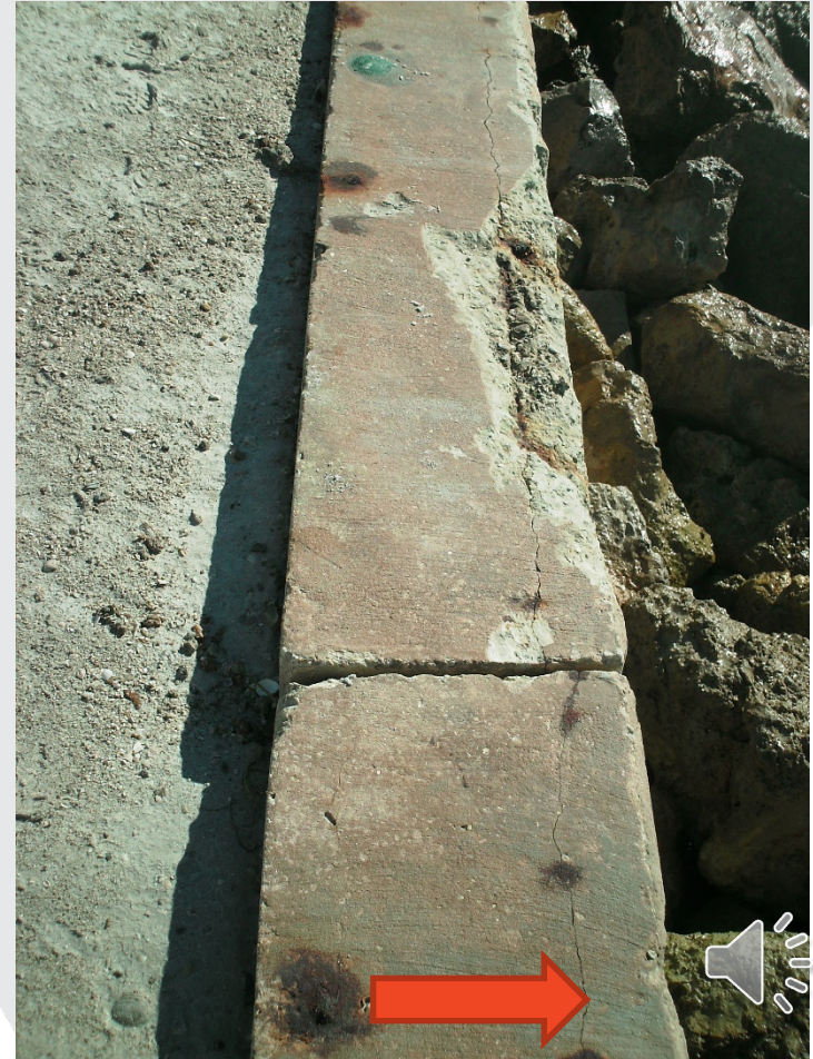
Gulf Coast Seawall
